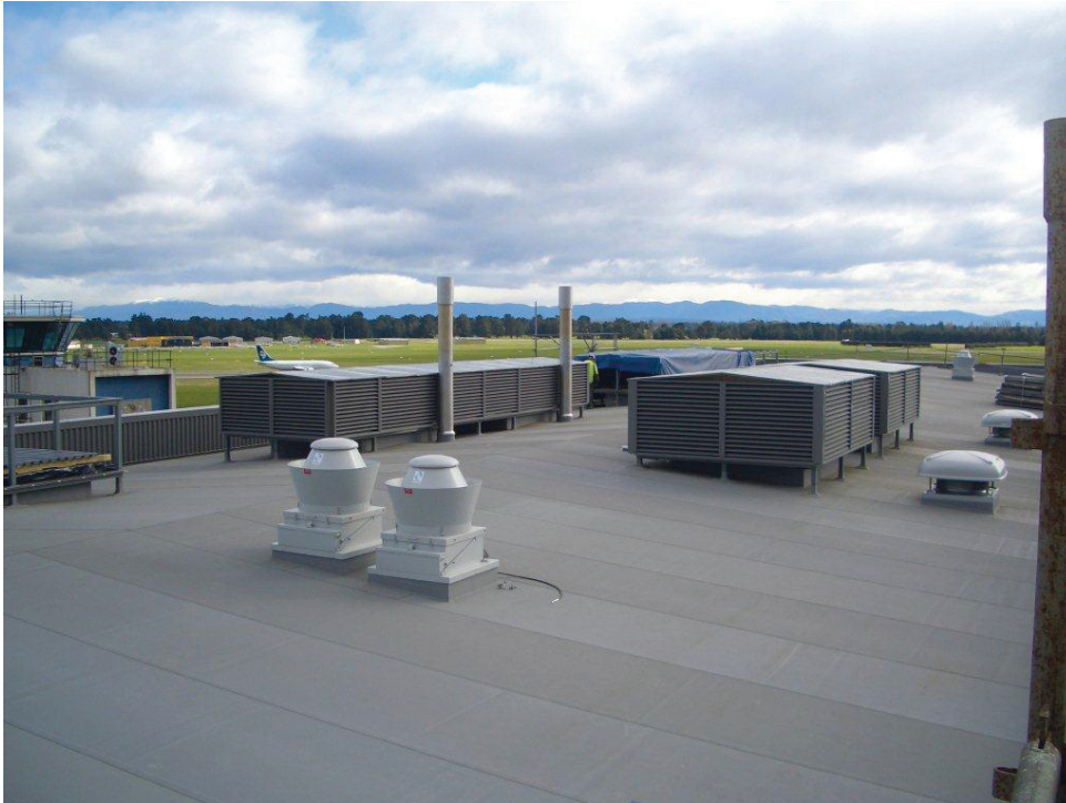
The new Christchurch Airport Terminal has been covered with 1.5mm Dove Grey Butynol.
