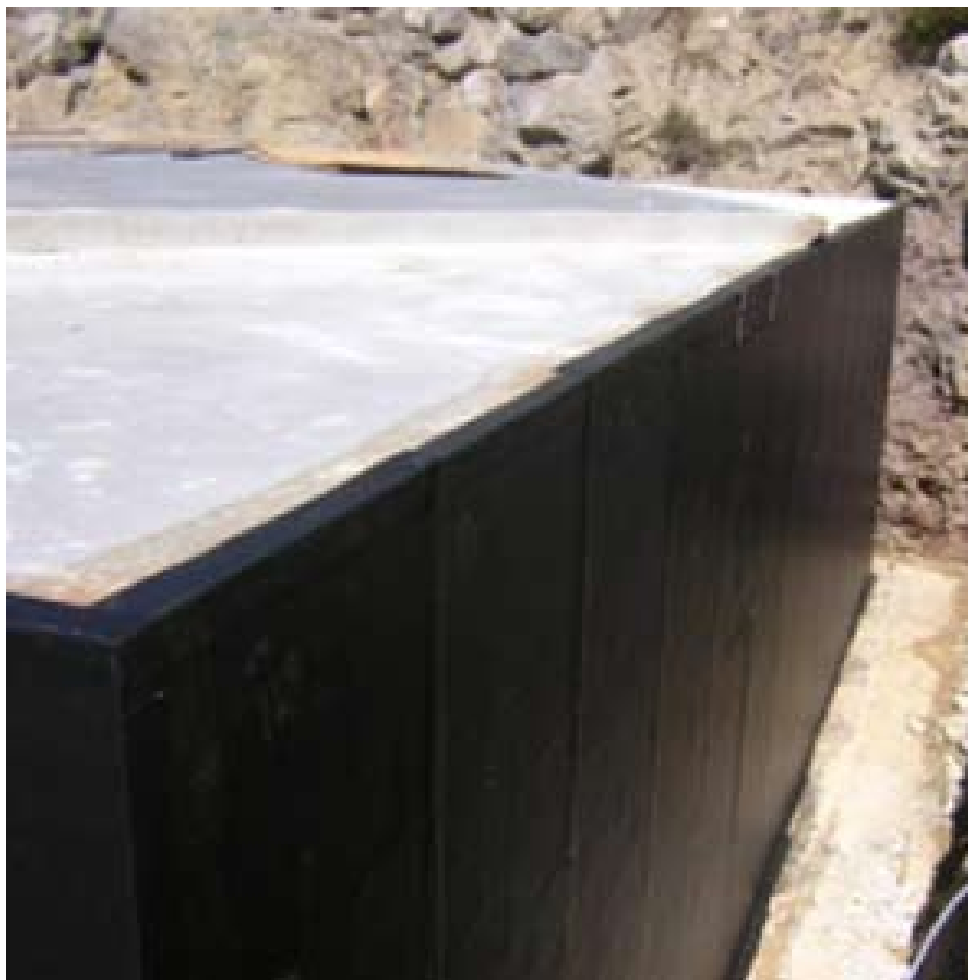
Typical waterproofing using Shelterseal 3000X
