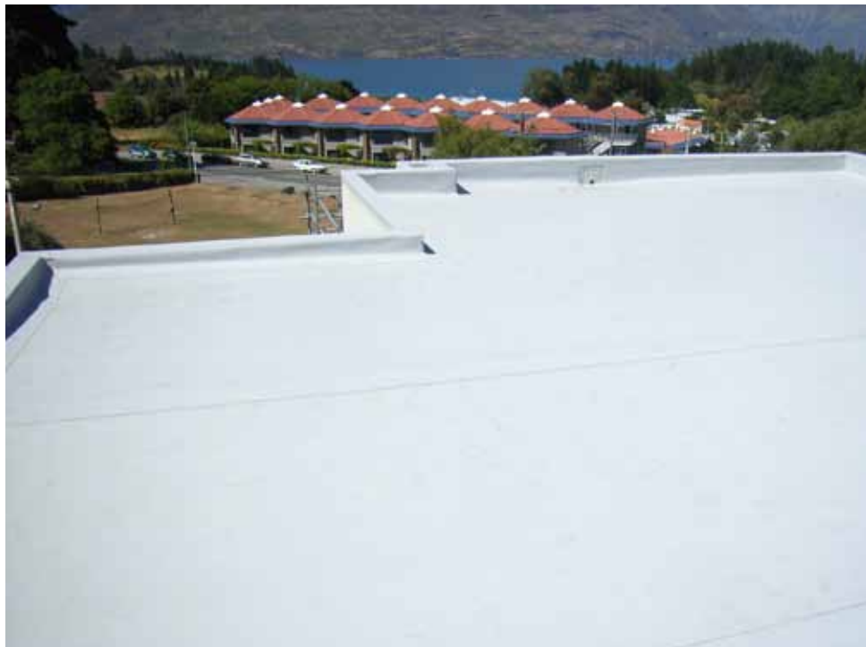
The roof of the Scenic Circle Aurum Hotel, Queenstown.
