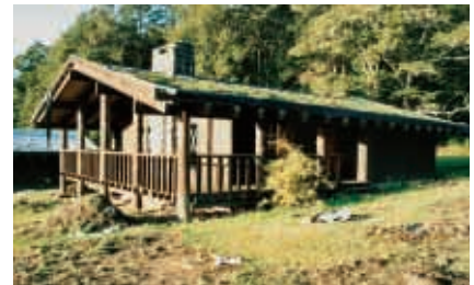
These chalets which form part of Takaro Lodge at Te Anau are a fine example of living roofs using Butynol as the waterproofing membrane
