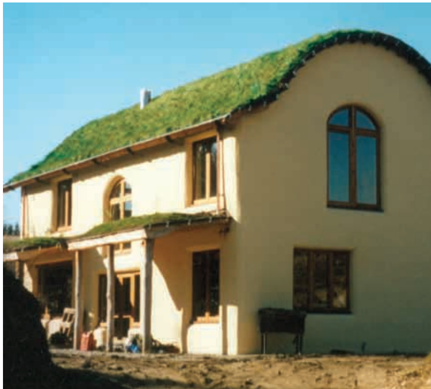
These chalets which form part of Takaro Lodge at Te Anau are a fine example of living roofs using Butynol as the waterproofing membrane
