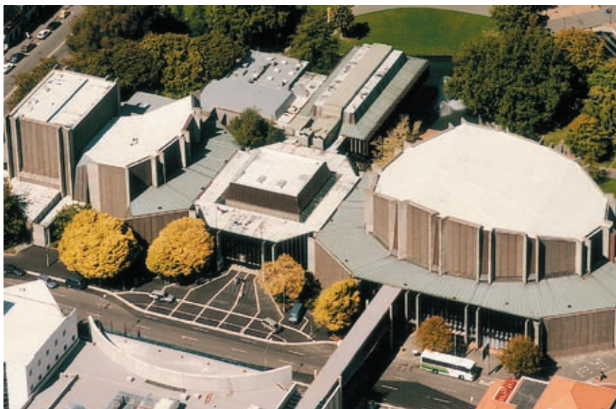
Current View of Christchurch Town Hall. 1 mm Butynol® Roof Membrane laid 1972.
