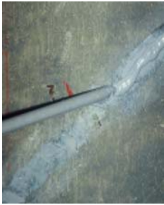
Capping cracks
