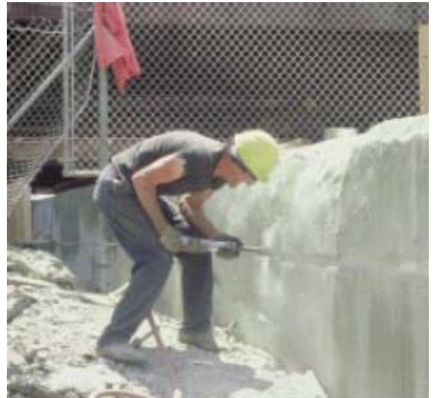
The capping material is ground off after the crack is repaired.
