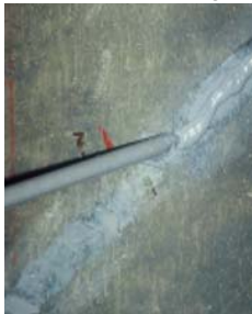
Capping cracks
