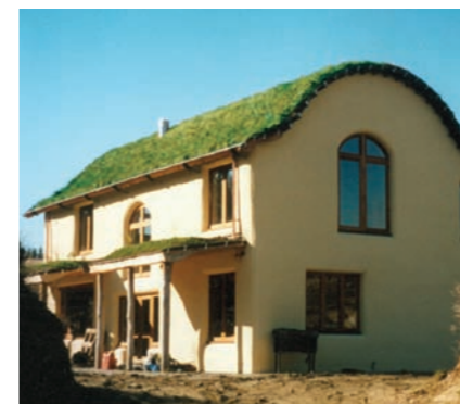
The McGregor House in Wanaka, by Richard Wilden Design, Dunedin has a unique bell shaped green roof.
