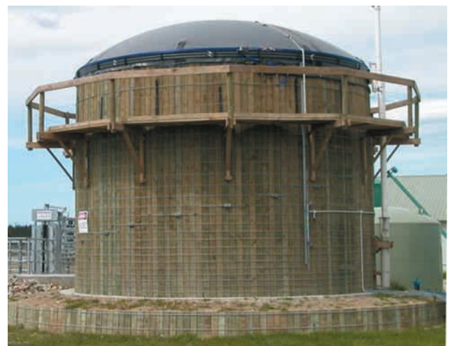
Digester tank with biogas inflated Butynol roof membrane
