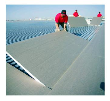
ARDEX Polyiso Board is the perfect thermal insulation roofing option for a variety of projects including;
