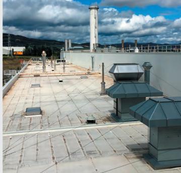
First UltraPly TPO roof in Europe (Pamplona, Spain). Sampling done in July 2019, 20 years after installation .
