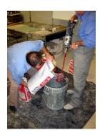
d. When adding the lightweight aggregate, the blades of the "ribbon type "mixing paddle must be visible to ensure that the vortex action of the mixing paddle effectively draws the aggregate (this is particularly important with the SL Grade Polystyrene Bead) into the mortar to blend and coat the aggregate and provide even distribution of it throughout the mix.
