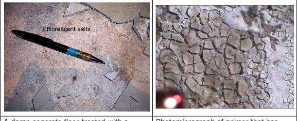
A damp concrete floor treated with a reactive silica based treatment that has developed severe efflorescent salts deposits. The smoothing cement has debonded off the powdery surface.
