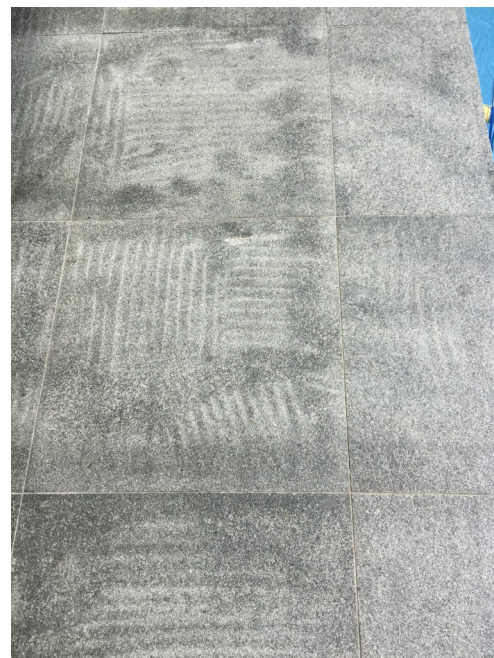
Figure 12. A mafic rock ('basalt, dolerite or diorite') displaying striping as a result of poor and incomplete contact coverage. The adhesive has altered the properties of the rock changing its porosity.
