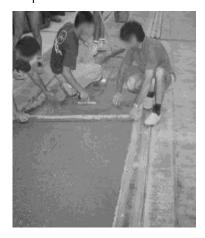
The poured material can be roughly shaped by scraping with a trowel after initial set, or once the filled leveller has cured, it can be diamond ground as required.
