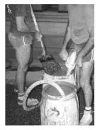
Mixing is performed with a high speed mixer such as a drill fitted with an ARDEX mixing paddle. Normal mixing is done for 2 minutes, and then the aggregate/sand is added and mixing continued till the aggregate is wet out.
