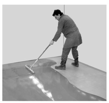
6. The floor spreading tool is used to smooth out the surface after it has been raked, or spreading the poured cement if the surface is too irregular to use the thickess rake
