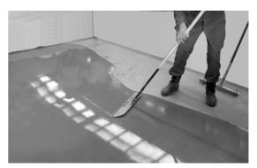
7. The last pass against a door or wall is done by pulling the tool along and walking backwards to the exit point, which is then finished with hand trowels.
