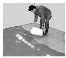
Pour the smoothing cement whilst walking along, and always apply to the wet working edge.
