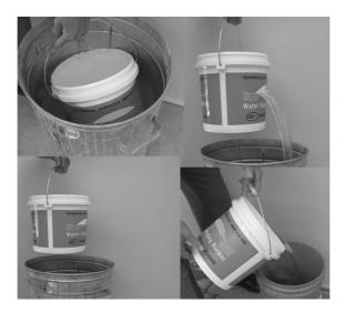
2. Take a bag of the floor leveling cement and pour it into the mixing bucket whilst at the same time commencing to mix with the power stirrer. *Note that hand mixing is not satisfactory and will not mix the product properly.*
