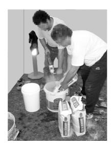
By cutting the bag to produce a flap, it is possible to minimise the amount of dust produced during the pouring and mixing process.
