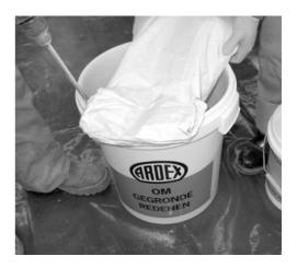
3. The material shall be mixed for two minutes in total and the paddle should be scraped around the sides to break up any adhering dry material.
